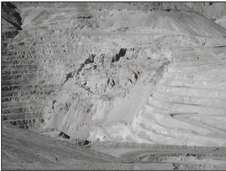
FIGURE 23.2 Examples of pit slope failure mechanisms in mined-out pit. The larger failure is probably because of structural controls; the effects of smaller raveling failures can be seen on some of the benches as they are filled with finer materials.
