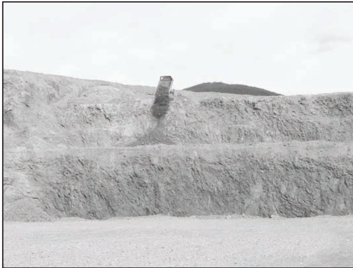
FIGURE 20.4 End dumping material to backfill a portion of the Surprise pit at the Zortman–Landusky mine, Montana
