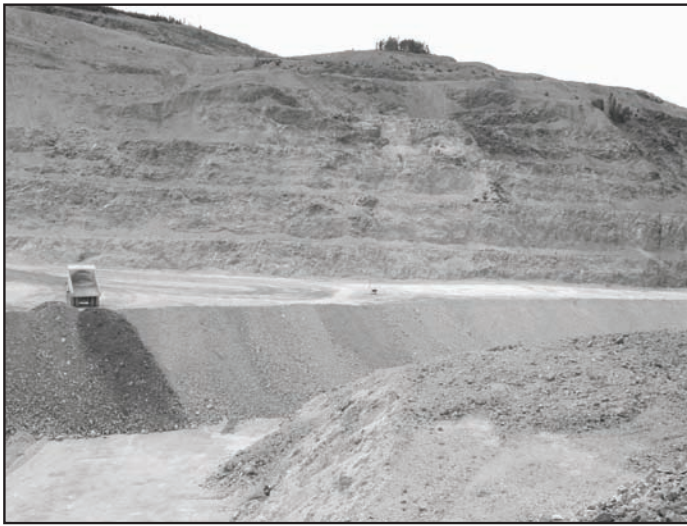
FIGURE 20.6 OK-Ruby pit backfilling to cover sulfide-bearing rocks in pit floor, Zortman–Landusky mine, Montana
