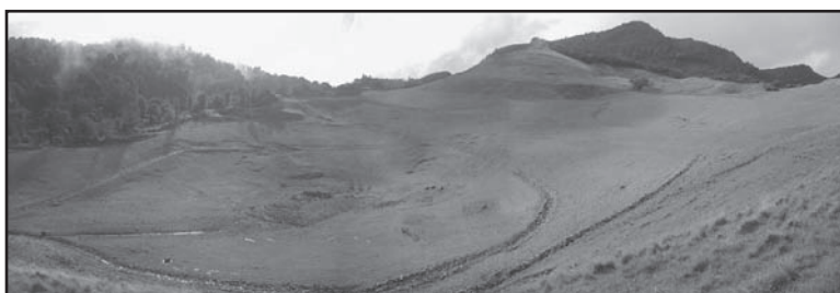
FIGURE 20.13 The backfilled and rehabilitated Golden Cross mine, New Zealand, 2002. Notice the extensive surface drainage network.
