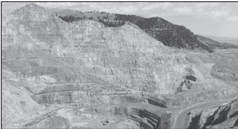
FIGURE 20.3 An example of the structural and lithologic complexity at the Golden Sunlight mine, Whitehall, Montana. Each of the structural elements must be evaluated and characterized for groundwater flow potential as one evaluates potential backfilling issues.
