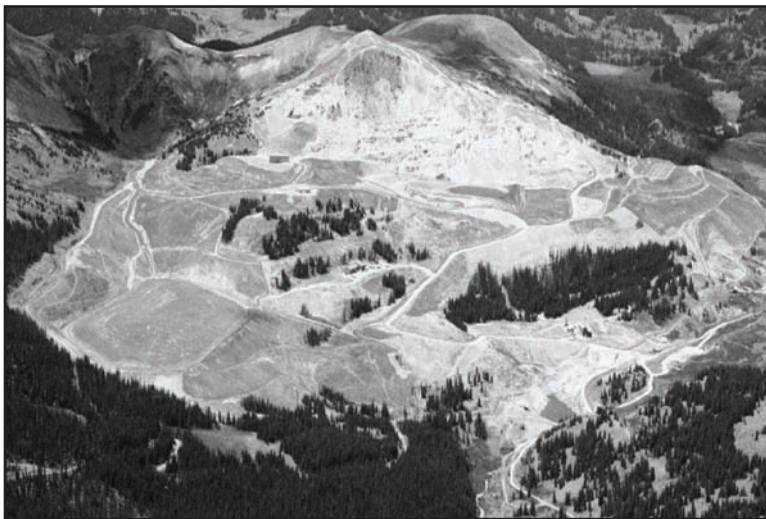
FIGURE 20.15 Summitville mine, Colorado, after reclamation. Notice the minor use of pit backfill against the open cut face.
