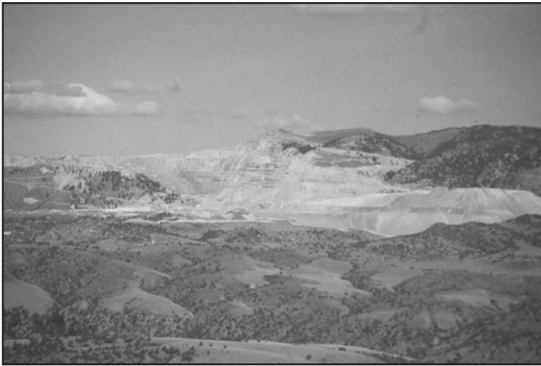
FIGURE 20.2 Golden Sunlight mine, Whitehall, Montana, showing pit highwalls and typical waste rock terrace features
